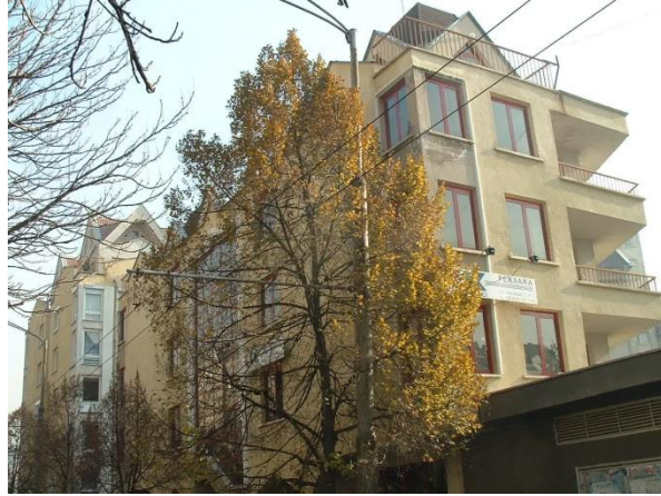
FIGURE 3. E-N Façade before re-habilitation
