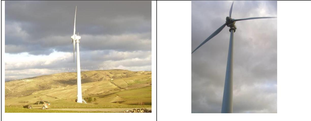
**FIGURE 3.** Towers with tubular structures.
