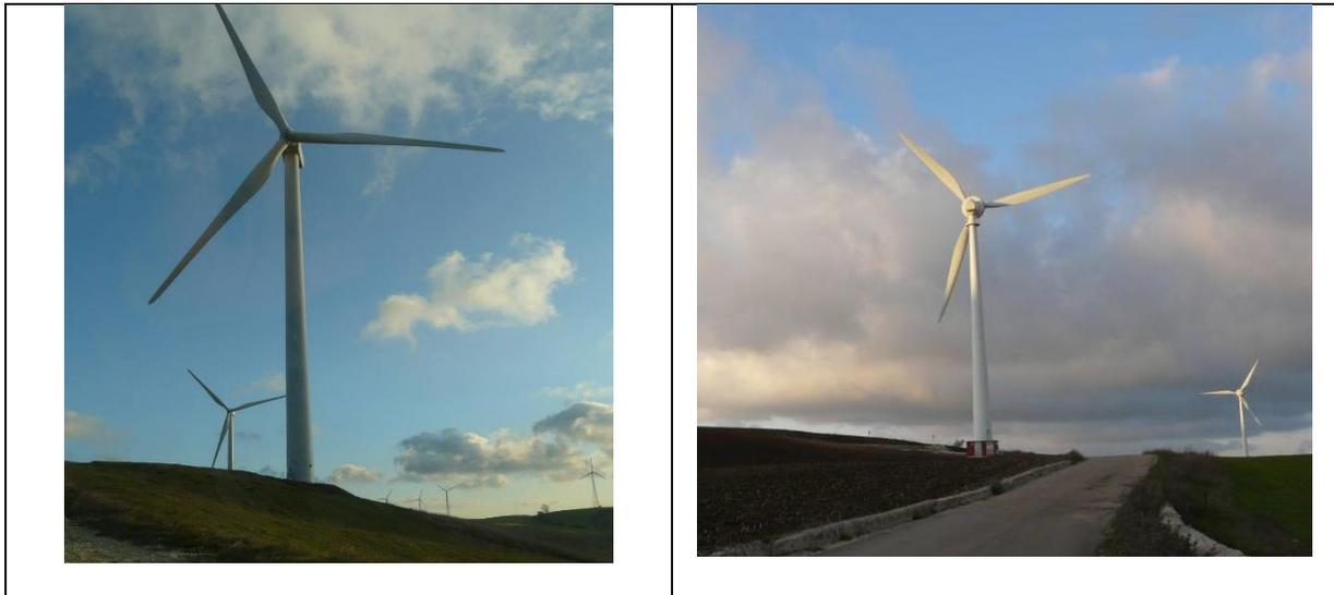
**FIGURE 4.** Towers with tubular structures.
