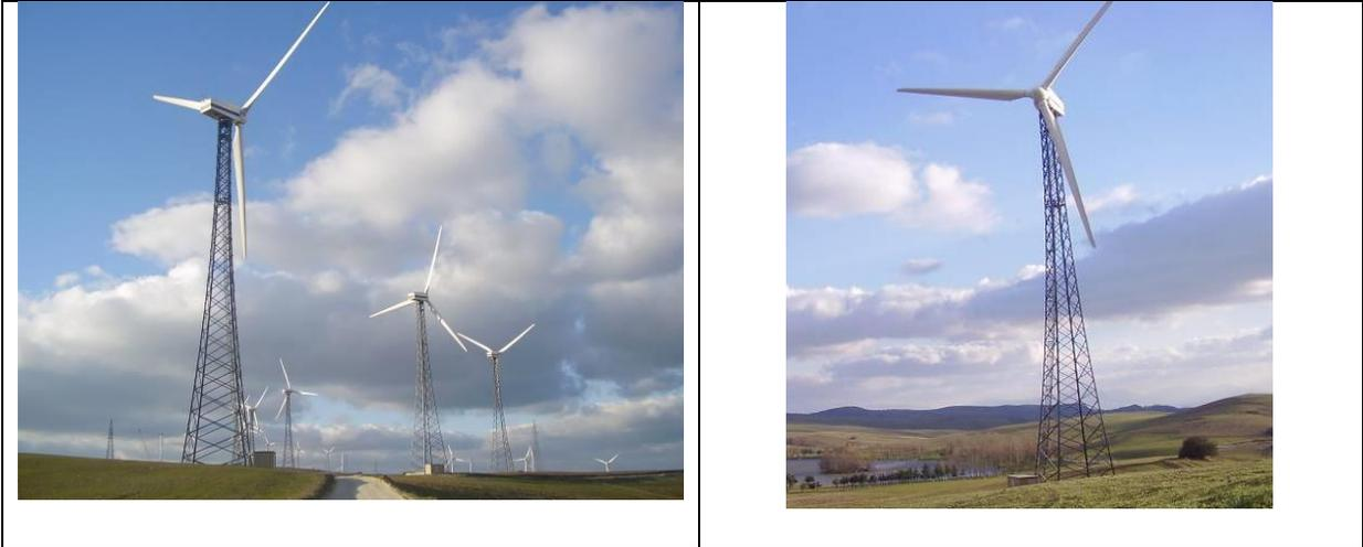
FIGURE 2. Towers with reticular structures.
